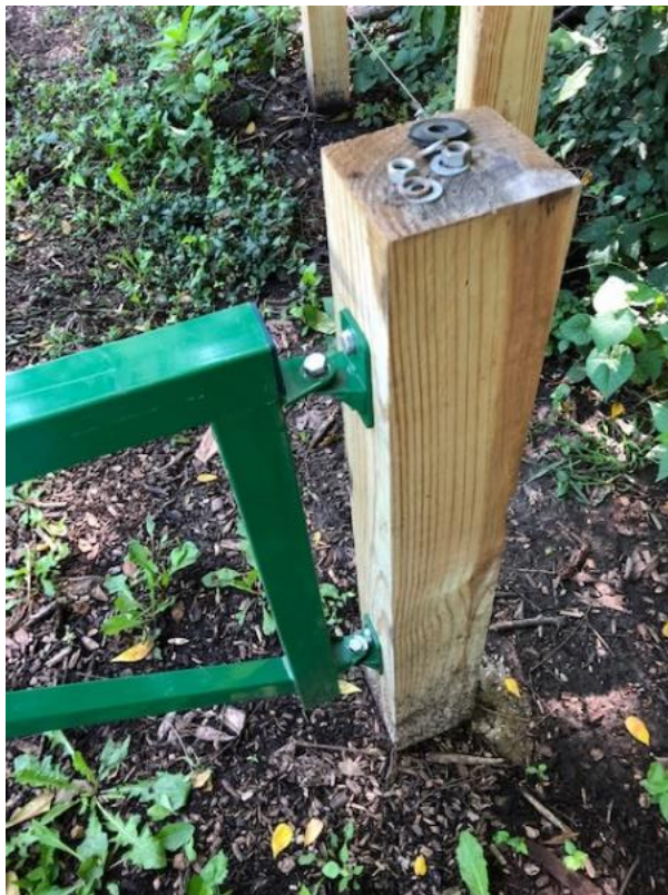
Installed new gates, September 11, 2019
