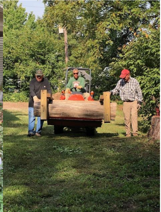
Installing bench, September 19, 2019
